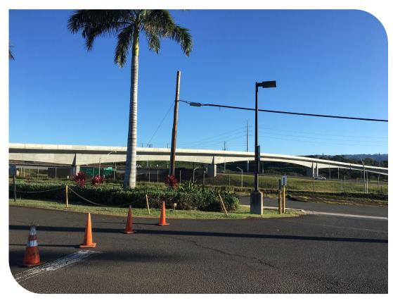
Bridge in Hawaii, part of the Honolulu Metro Rail system – outfitted with 3 Hyperion systems connected to 153 sensors for structural monitoring
